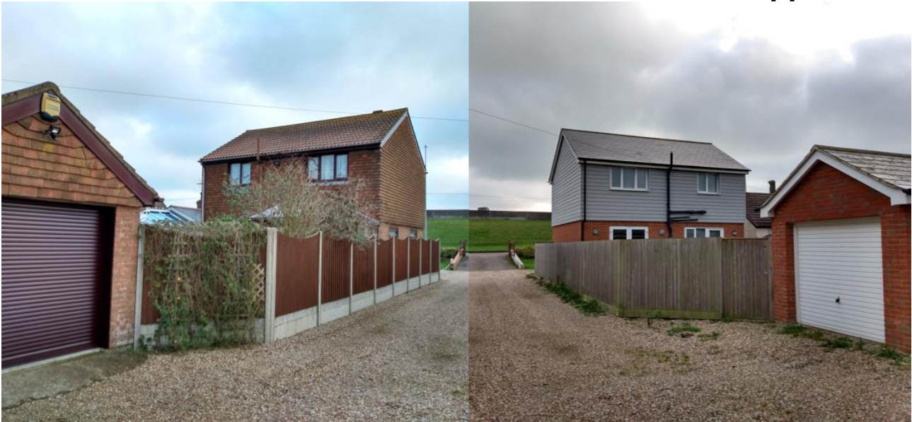
Photo 4: Rear of 1 and 2 Willop Close
